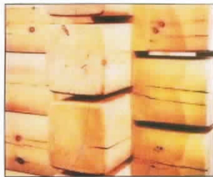
SADDLE-NOTCH CORNERS look traditional but don't shed water as well.
