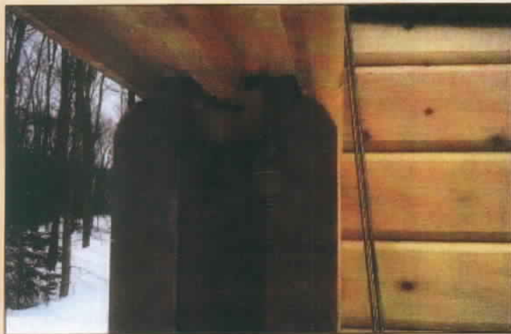
REINFORCING OPENINGS for windows and doors with steel bars (shown left) is key in a frame of shifting logs.
