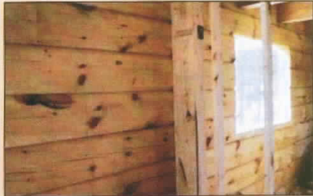
REINFORCING OPENINGS for windows and doors with steel bars (shown left) is key in a frame of shifting logs.
