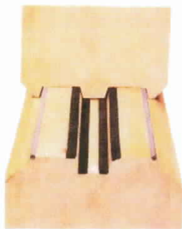
BETWEEN LOGS , foam and butyl tape form a tough, durable seal.
