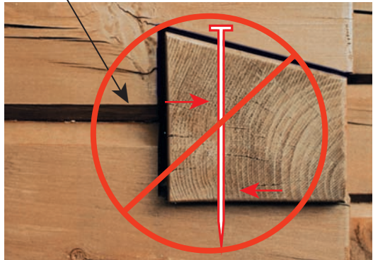
Competitor's corner will shrink toward the nail (red arrows)
